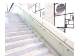
Installation of bar (A-PLACE Bashamichi)
