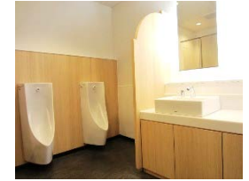
Renovated toilet room (A-PLACE Shinagawa)
