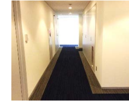
Improved interior finish of sharing corridor (A-PLACE Shibuya Konnoh)
