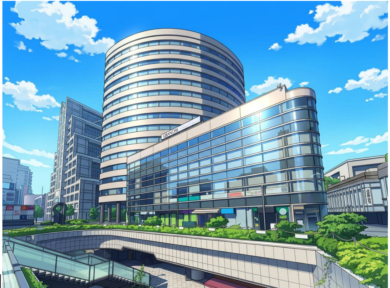
Aoyama Oval Building
